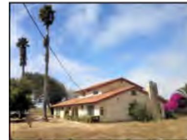
Existing residence on property
